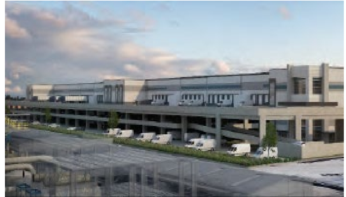
Trammel Crow will develop a 2-story 695,000 square foot light industrial warehouse on Terminal 106
